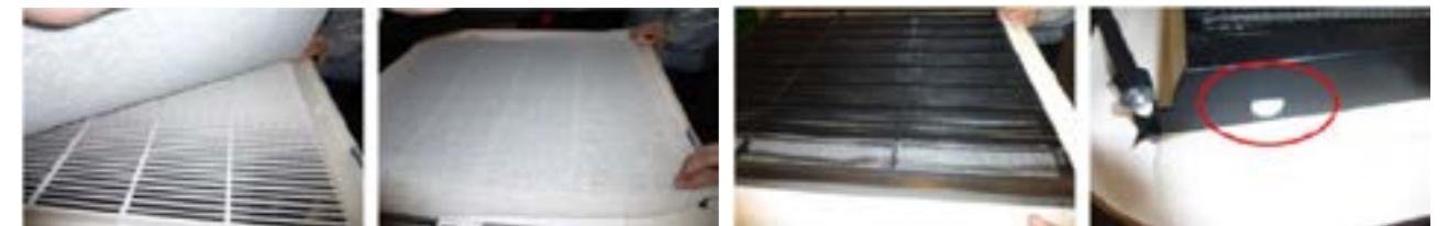
1. Set the pre-filter inside of grill cover.
